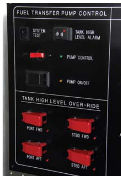
Primary fuel filters and priming systems are located inboard of each engine. (top) Fuel transfer controls and override switches are clearly labeled and easily accessed. (bottom)
